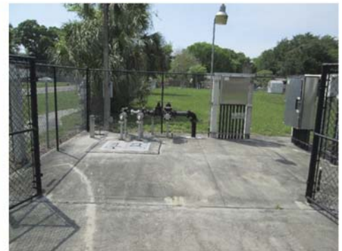
Figure 6. Lumsden No. 5 Pump Station: “Before” Images Showing Old Suction Lift Pump Station With Discharge Force Main (white polyvinyl chloride) Exiting Through Block Wall (top); “After” Rehabilitated Pump Station (bottom).
