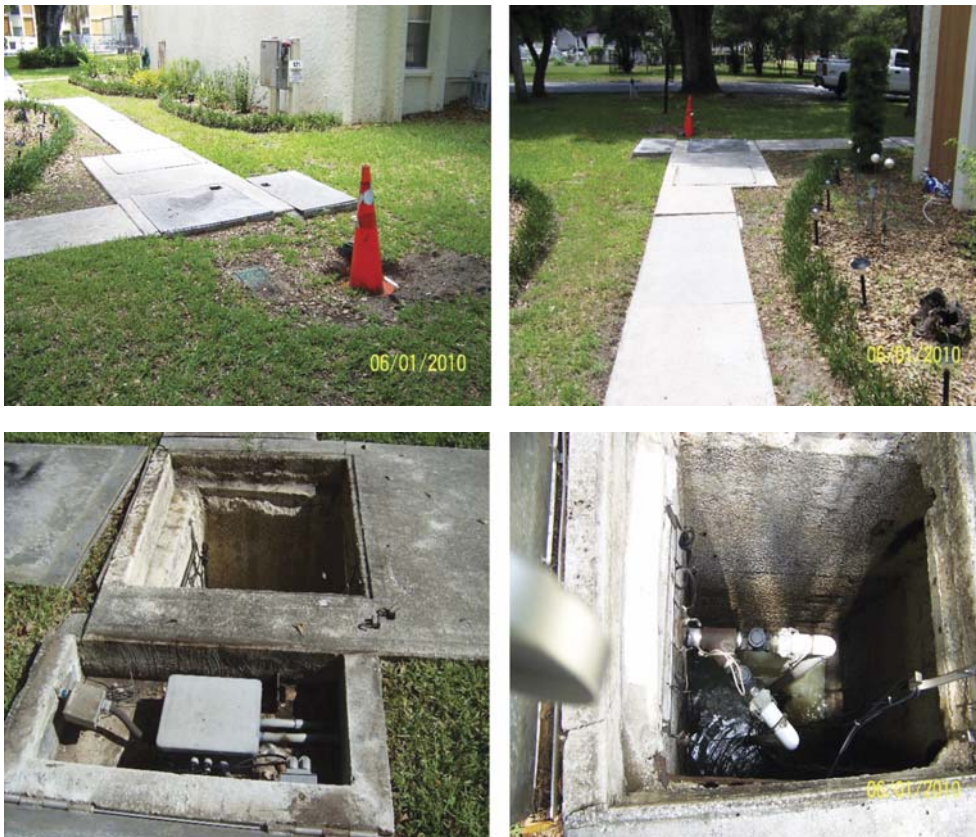
Figure 4. "Before" Images of Pinewood Pump Station (clockwise from upper left): Old Pump Station Overview Looking East With Control Panel in Background; Old Pump Station Looking West; Pump Station Wetwell and Electrical Vault; and Looking Into Wetwell.
